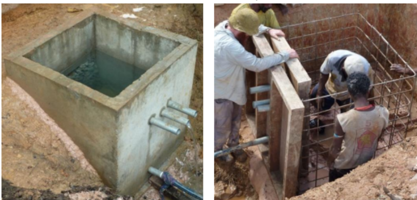
Figure A5: A spring box being constructed.
