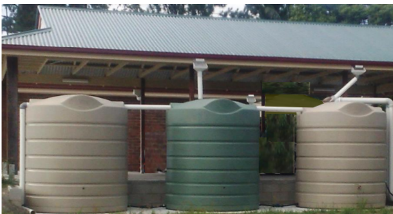
Figure A7: A typical roof drainage and rainwater tank collection system arrangement.
