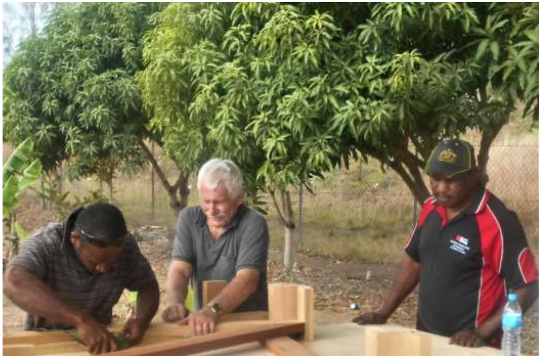
Practical building skills on-the-job mentoring, Papua New Guinea
