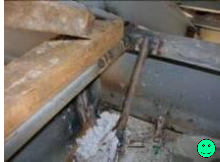
Welded Reinforcement - Thailand
