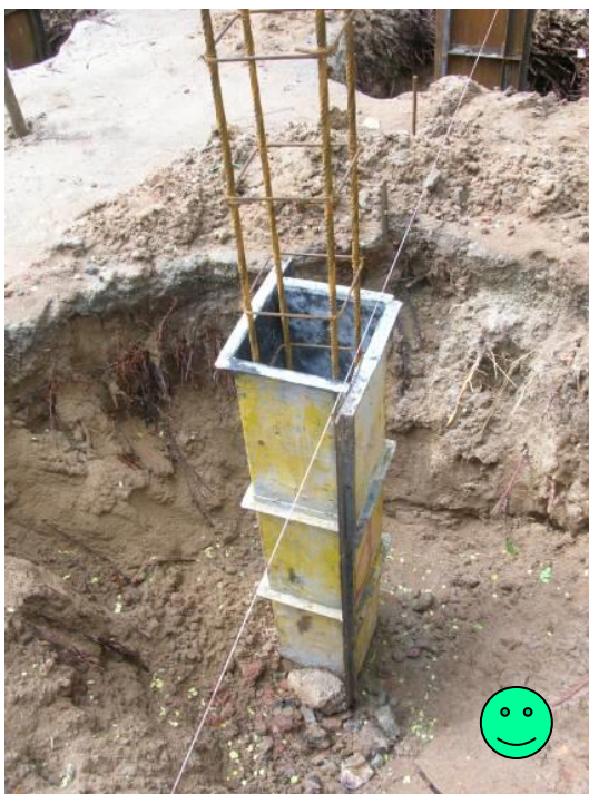
Pad Footings and Column Reinforcement India (Villupurum)
