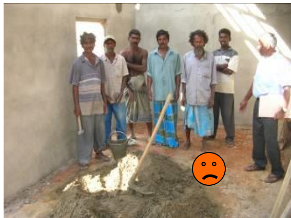
Unreinforced concrete slab-on-ground Sri Lanka (Trincomalee)
