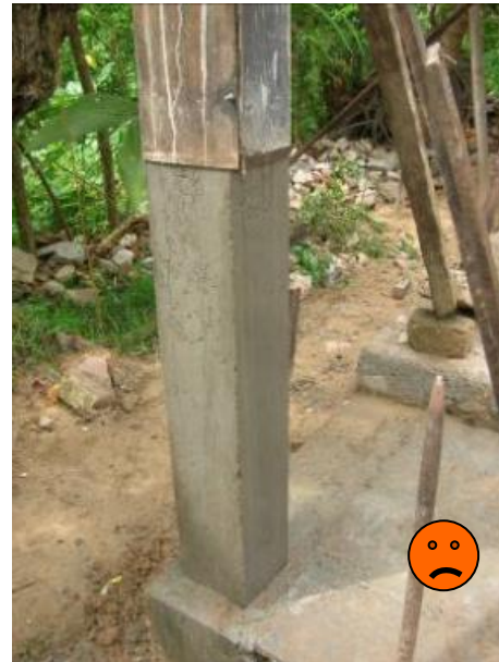
No ties between columns and masonry – Sri Lanka (Galle)
