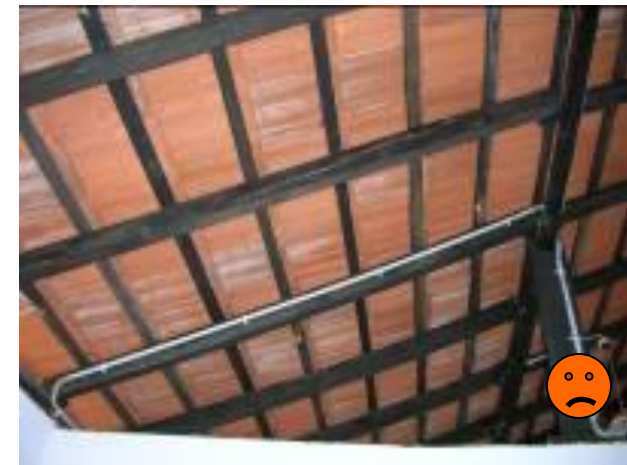
Tiles not tied down – Sri Lanka
