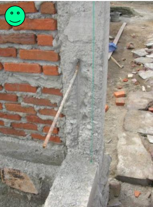
Brick to Concrete Columns Indonesia (Aceh)
