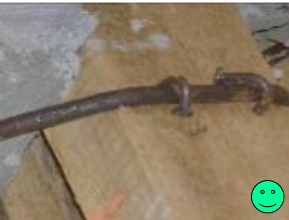
Bent reinforcement – Aceh
