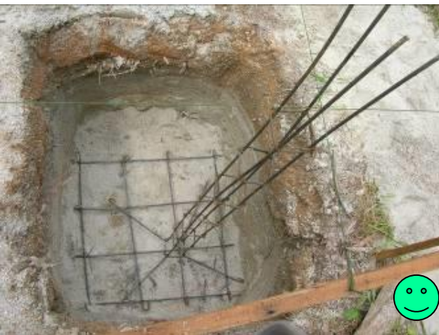
Pad Footings and Column Reinforcement Thailand
