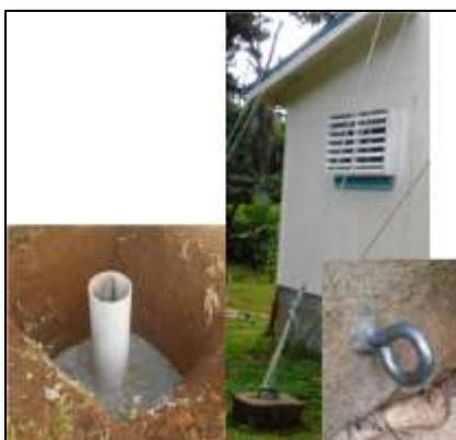
Cyclone Anchorages, Cook Islands, 2011-2012
