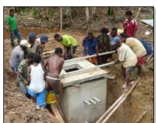
Spring Box, PNG, 2012 (with Emergency Architects)
