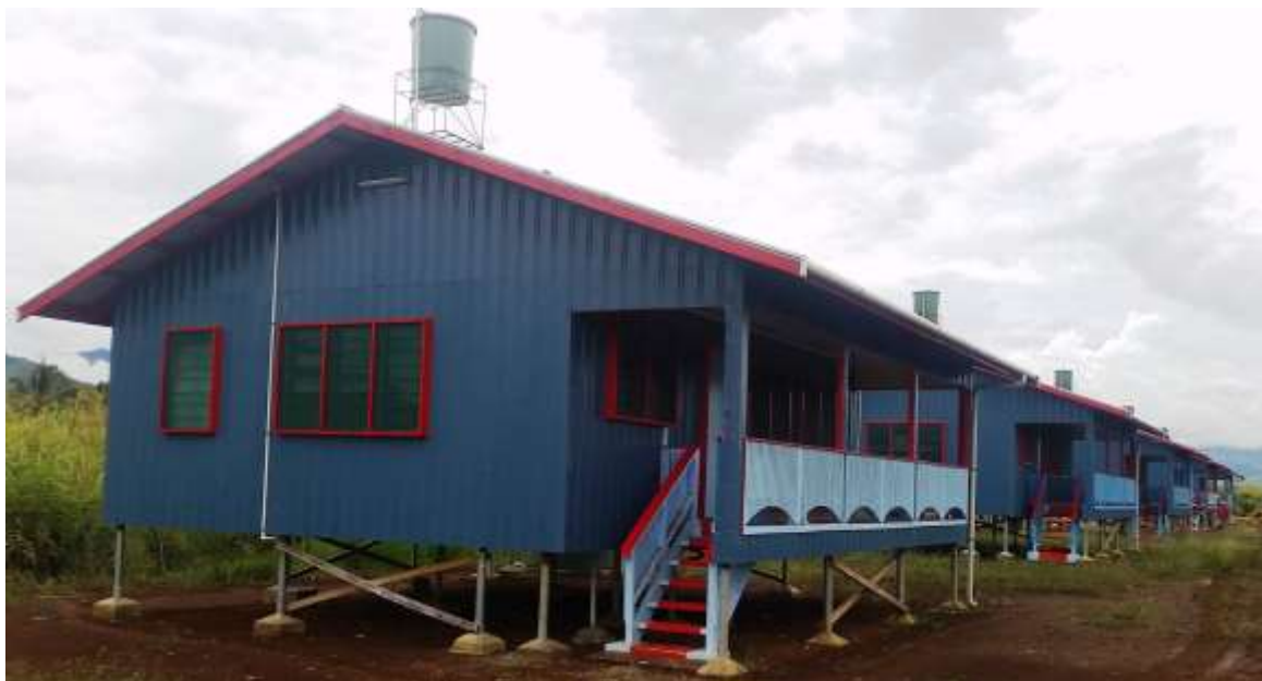
Five Police Houses constructed using the Partner Housing Australasia DANCER Building System at Baiyer River for the Government of Papua New Guinea.
