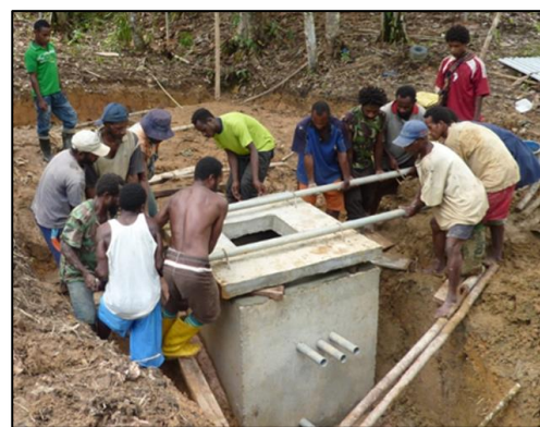
Spring Box, PNG, 2012 (with Emergency Architects)
