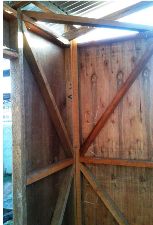
Braced Bolted and Built
