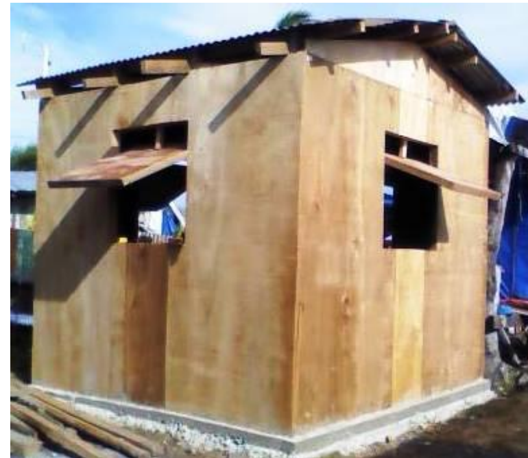
Rebuilding after Hurricane Haiyan
