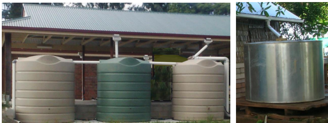
Figure A7: A typical roof drainage and rainwater tank collection system arrangement.
