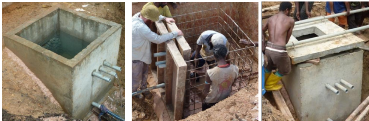
Figure A4: A spring box being constructed.
