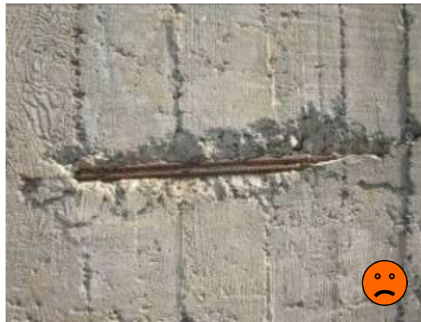
Concrete wall corrosion (Australia)
