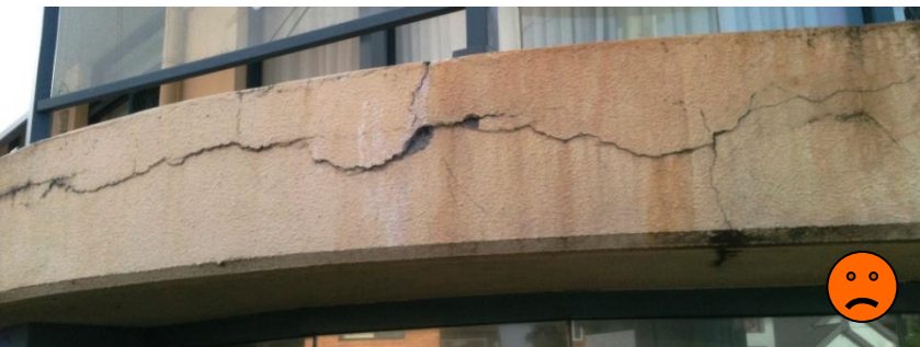
Concrete corrosion (Australia)
