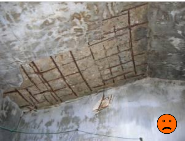
Suspended concrete roof corrosion (India)
