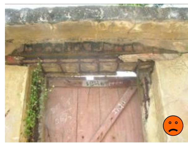
Concrete lintel reinforcement corrosion (India)
