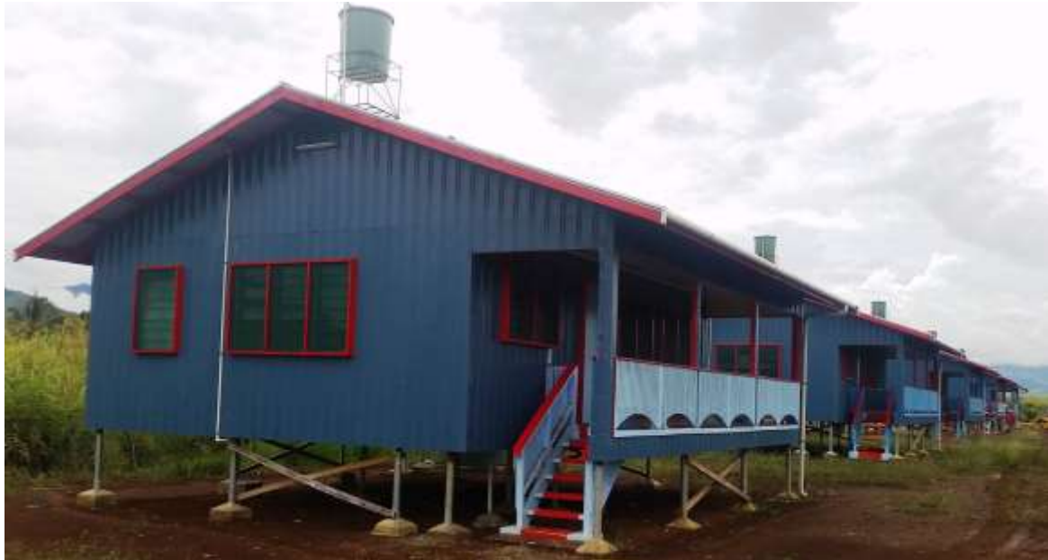
Five Police Houses constructed using the Partner Housing Australasia DANCER Building System at Baiyer River for the Government of Papua New Guinea.
