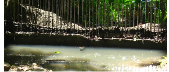
Vertical reinforcement for future extension
