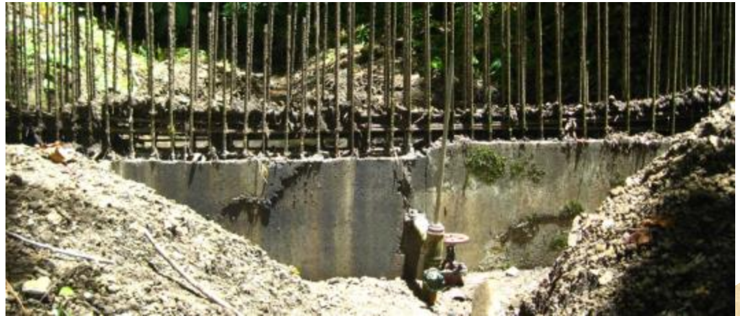
Vertical reinforcement for future extension
