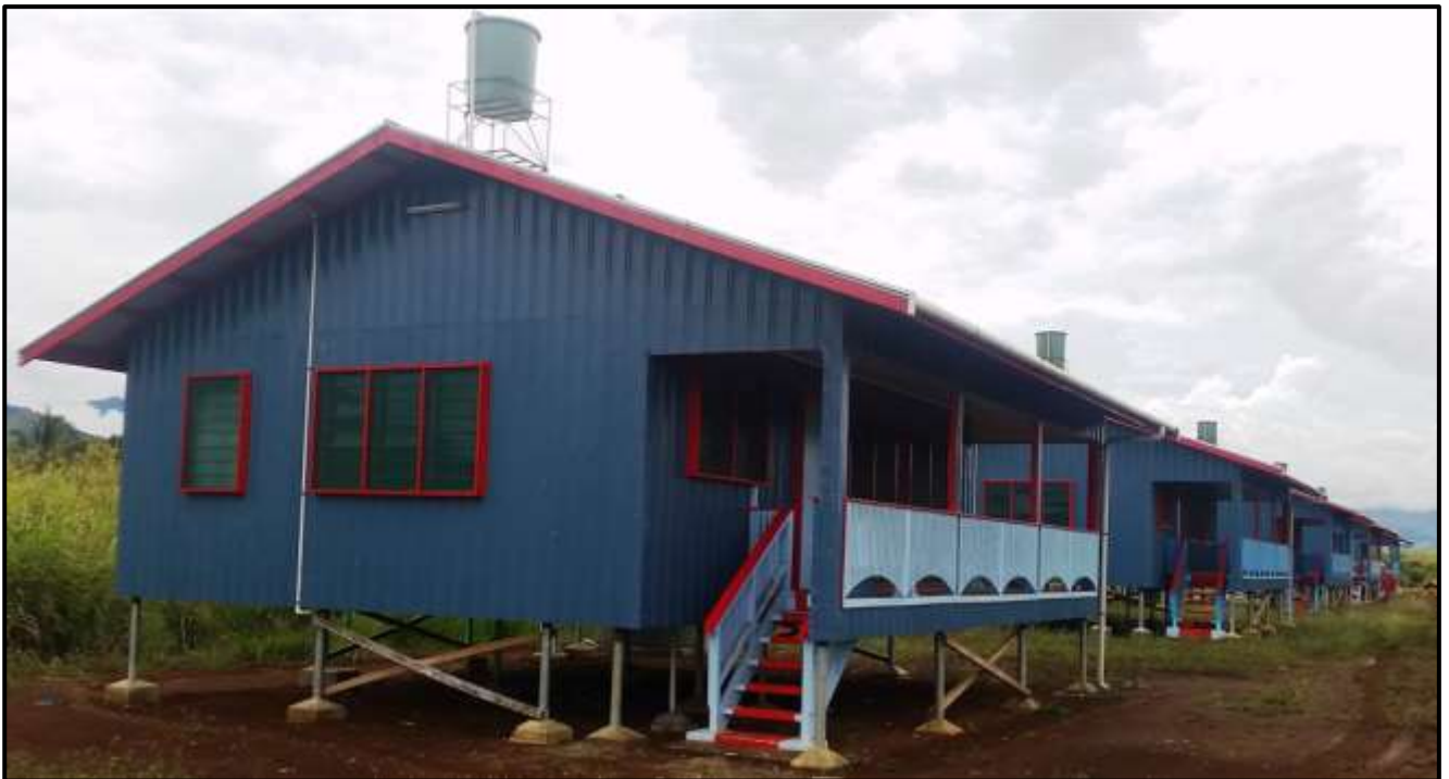
Five Police Houses constructed using the Partner Housing Australasia DANCER Building System at Baiyer River for the Government of Papua New Guinea.
