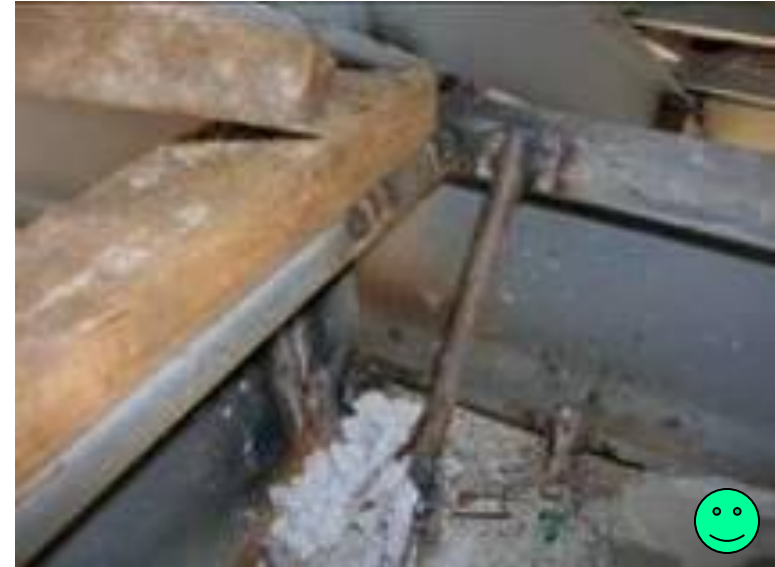
Welded Reinforcement - Thailand
