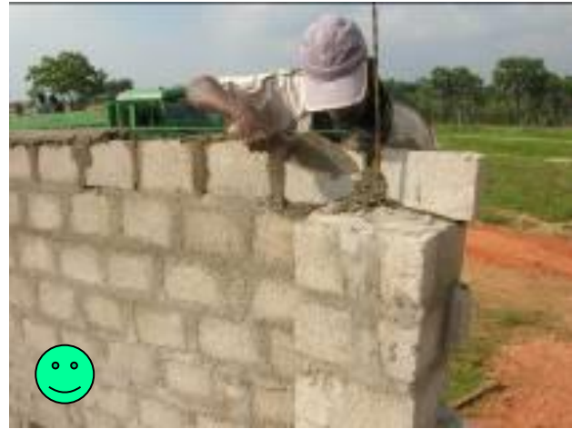
Bonded Masonry - Sri Lanka (Trincomalee & Batticaloa)
