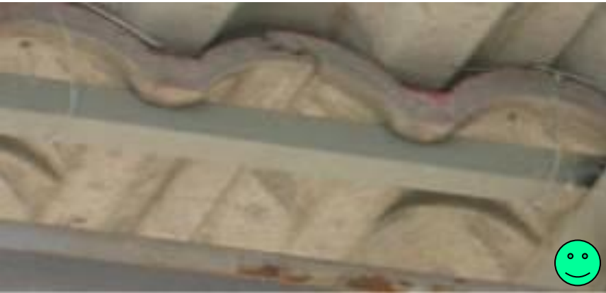
Tiles tied down – Thailand
