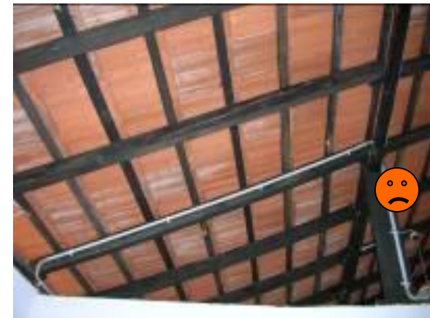
Tiles not tied down – Sri Lanka
