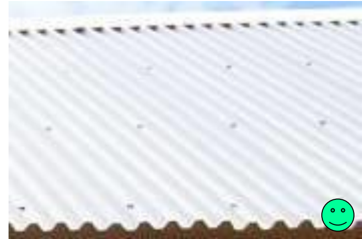
Roof sheeting tied down – Indonesia
