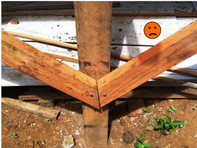
Bolts too close to the end of timber brace Papua New Guinea (Mt Hagen)
