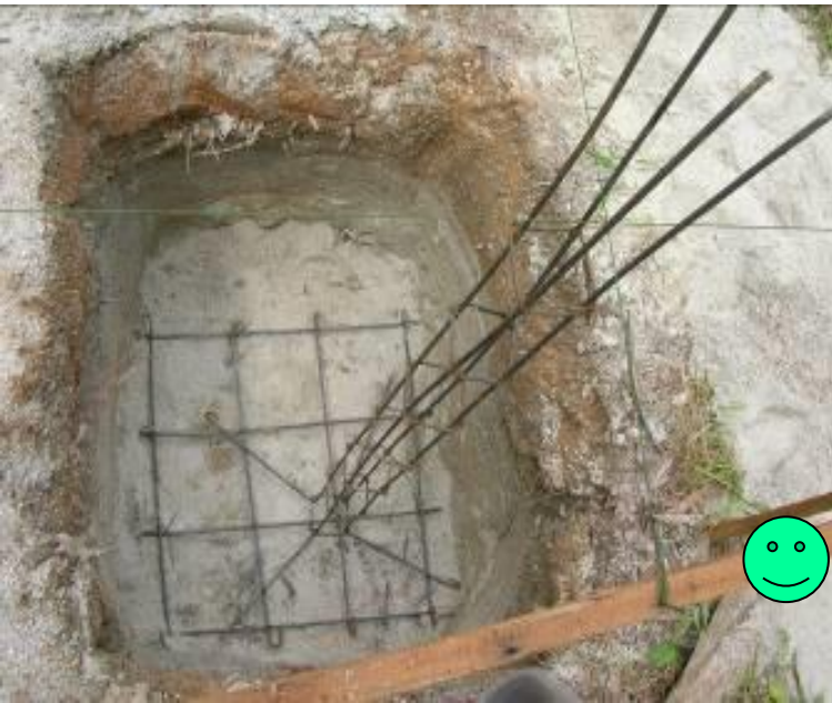
Pad Footings and Column Reinforcement Thailand
