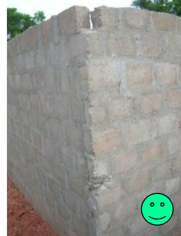
Bonded Masonry - Sri Lanka (Trincomalee & Batticaloa)
