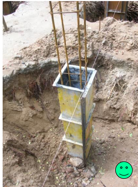
Pad Footings and Column Reinforcement India (Villupuram)
