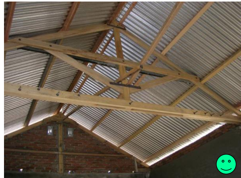
Framed Roof - Aceh
