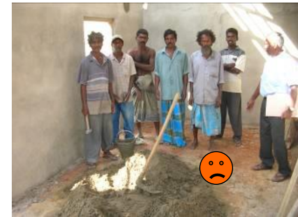
Unreinforced concrete slab-on-ground Sri Lanka (Trincomalee)
