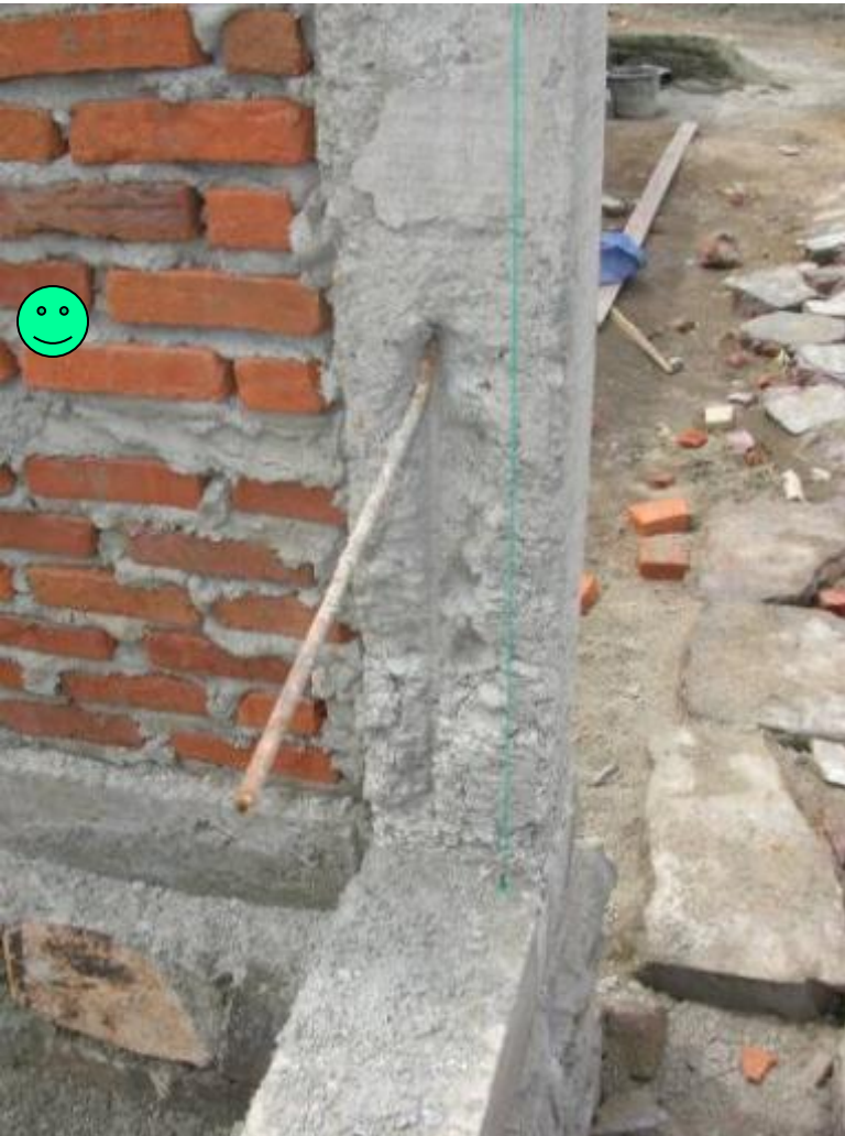
Brick to Concrete Columns Indonesia (Aceh)
