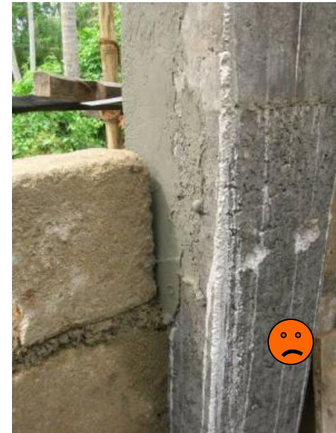
No ties between columns and masonry – Sri Lanka (Galle)
