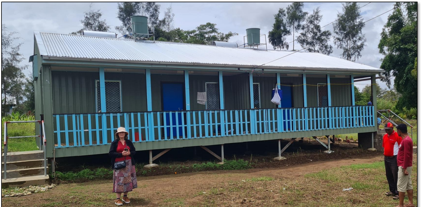
Kitip Secondary School, Staff Accommodation Duplex # 2, Completed September 2025
