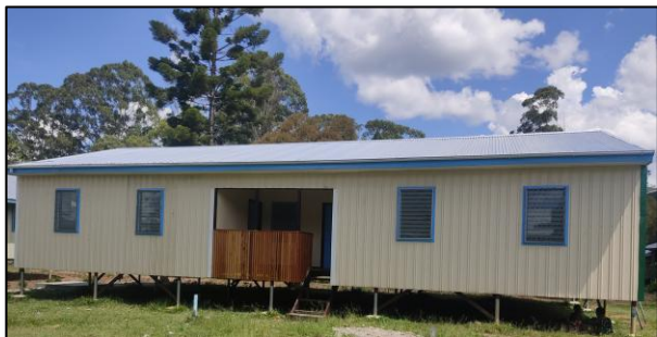
Kenembo School Two Classrooms and Office, 2023
