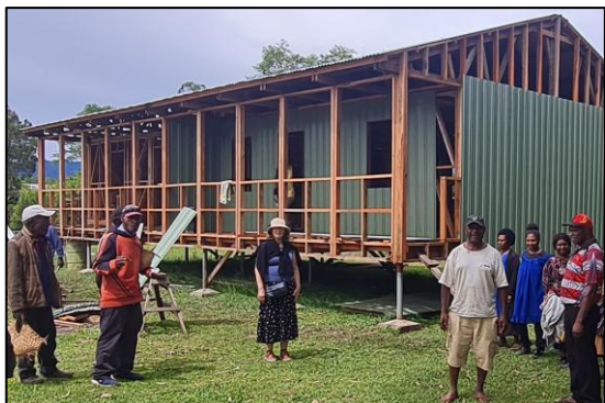
Kenembo School Duplex Staff House (under construction), PNG 2026
