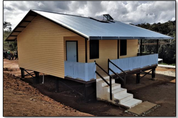
Kalolo Community Health Building, 2016
