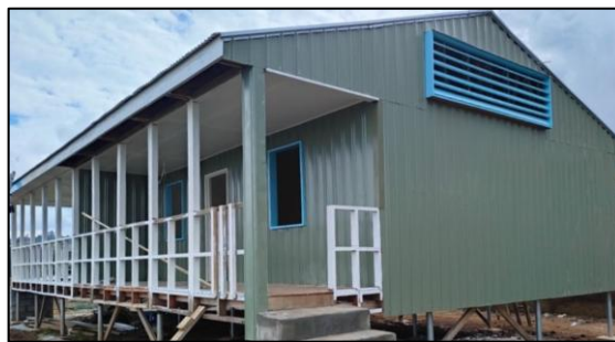
Kwip Dau School Duplex Staff House, 2024
