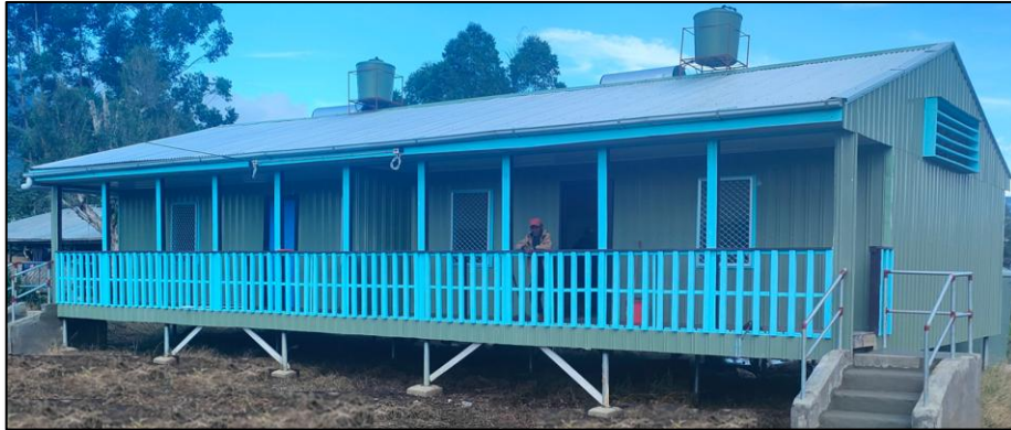
Kitip School Duplex Staff House No 1, PNG, constructed using the Partner Housing Australasia DANCER Building System
